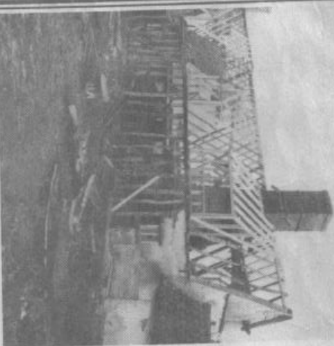
● This cottage near Denston was virtually derelict when the owner bought it for restoration. Below, a picture of the work in progress — work involved stripping its timber frame and replacing rotten timbers with sound ones.
